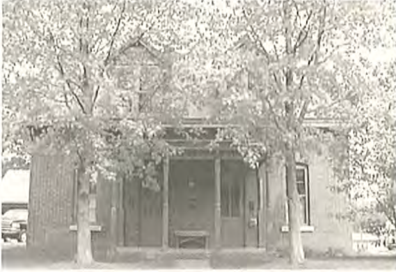
Henry Bauch House 1037 South 16 th Street
