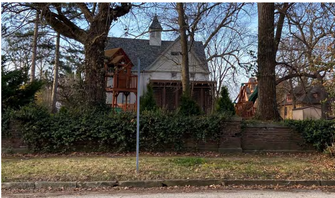
Hampshire Street View of 1636 Hampshire – 04/12/2022
