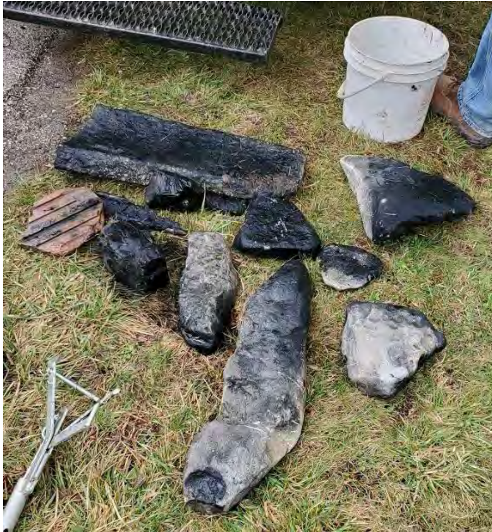
A sample of material pulled from a single manhole on the 30" interceptor at Cedar Creek (March '22).
