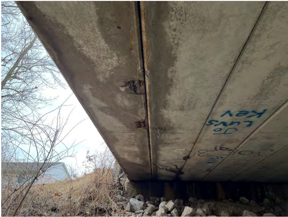
Photo No. 2 2/16/2022 Looking west at 1/3 span of south exterior beams
