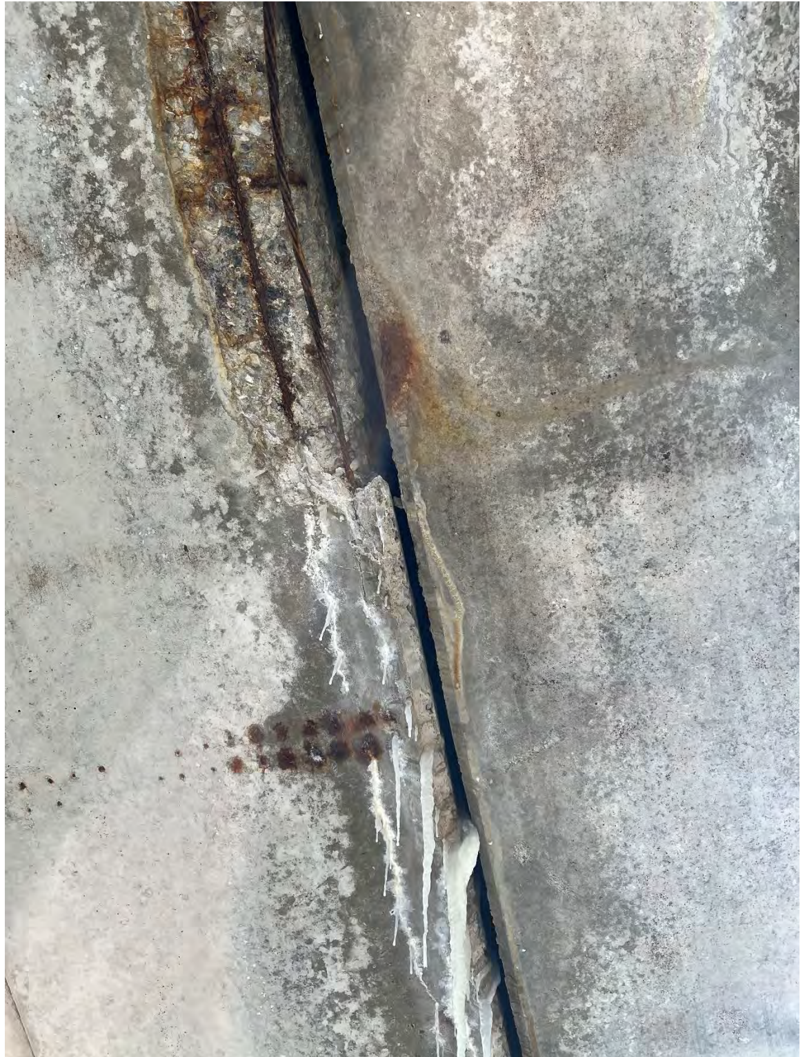
Photo No. 4 2/18/2022 Looking east along south exterior beams at mid-span
