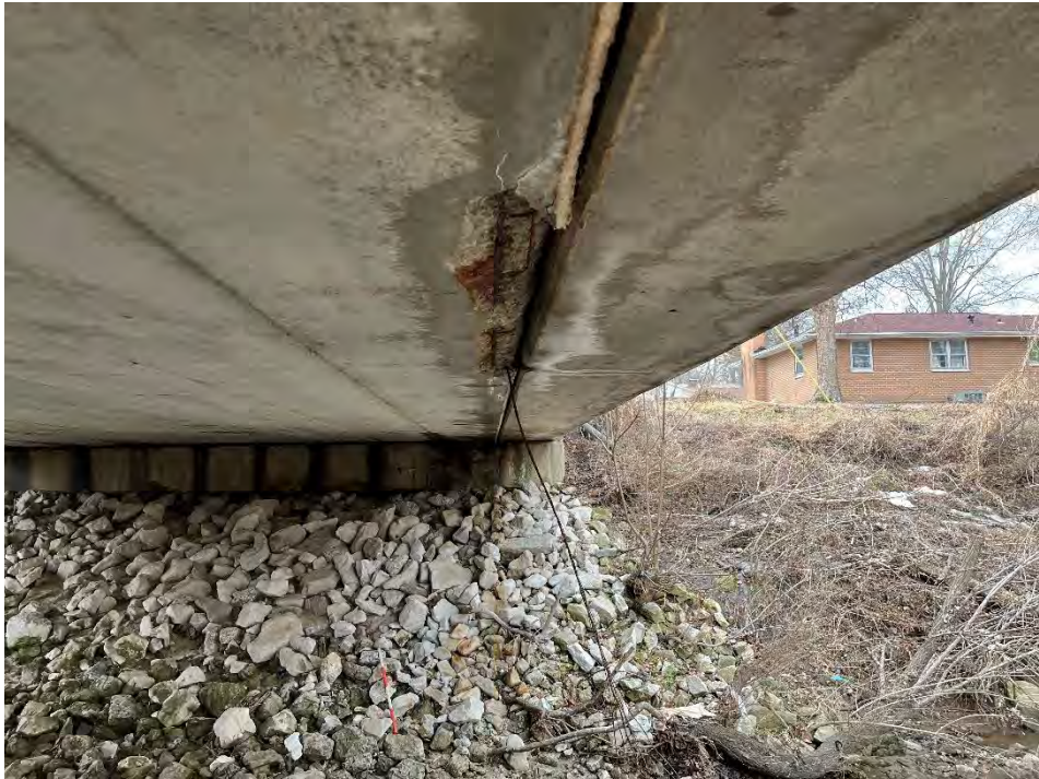
Photo No. 1 2/16/2022 Looking east at midspan of south exterior beams
