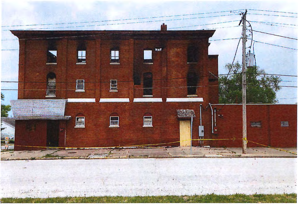
649 State Street Damage from Fire on May 18, 2022 Photos taken May 24, 2022
