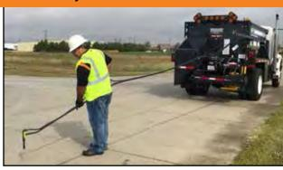
FP5 Pivot Tack System retains and supports the emulsion and air hoses, which supply the tack wand. The spring return retractor design prevents the hose from touching the ground and allows for 20 feet of spray wand coverage behind the patcher.
